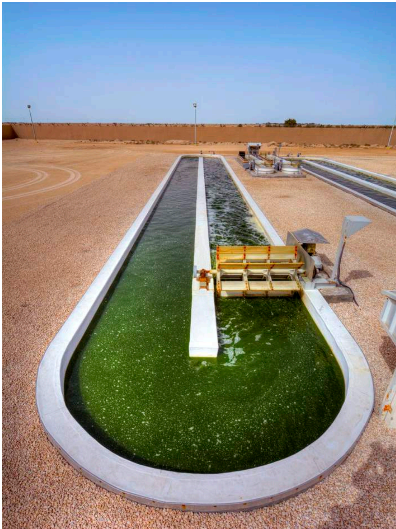
Open raceway pond constructed and operated as part of the Algae Biofuel Project with 25,000 litre capacity for outdoor cultivation of micro-algae under Qatar's climatic conditions
